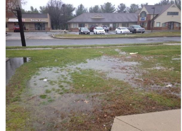
Stormwater is currently directed to the parking lot which connects to multiple storm drains. Parking spots on the northern side of the parking lot can be replaced with pervious pavement to capture and infiltrate stormwater. A rain garden adjacent to the building can capture, treat, and infiltrate roof runoff as well as reduce ponding on the property. A preliminary soil assessment suggests that the soils have suitable drainage characteristics for green infrastructure.
