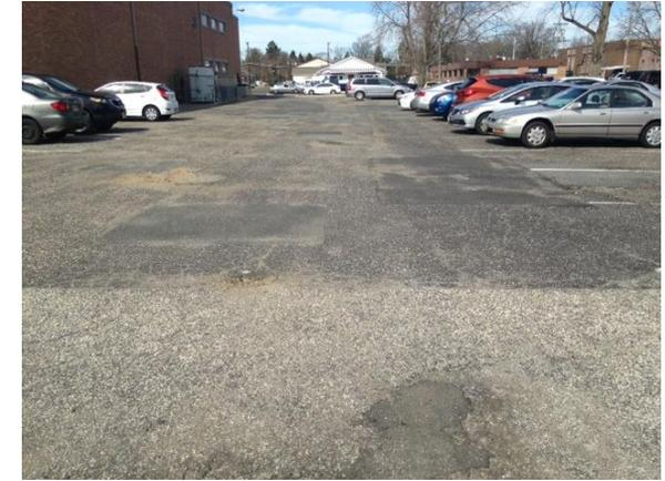
Stormwater is currently directed to a parking lot which connects to multiple storm drains. Parking spots on the west side of the parking lot can be replaced with pervious pavement to capture and infiltrate stormwater. A preliminary soil assessment suggests that the soils have suitable drainage characteristics for green infrastructure.
